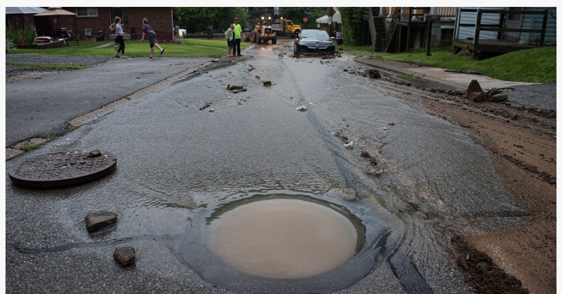
Clean-up from aftermath of a wet-weather event causing localized flooding and sewer overflows with legacy devices unable to locate sources of infiltration.
