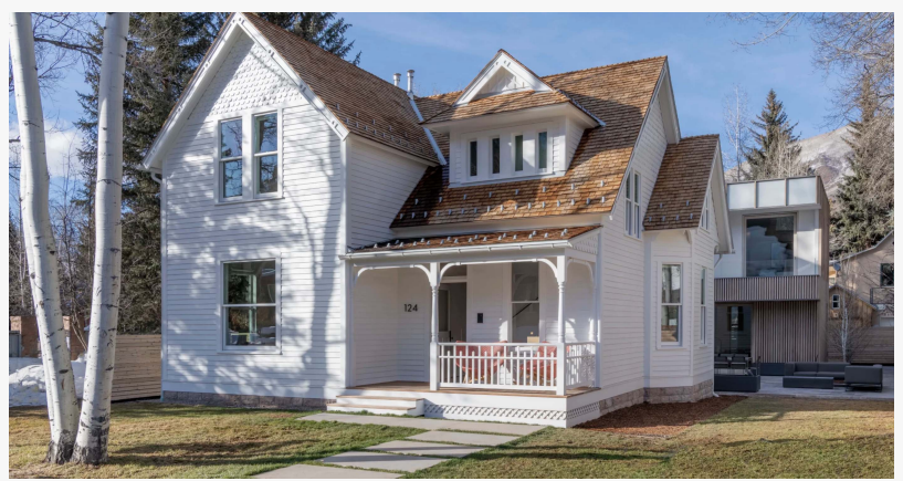
Exterior of 124 W Hallam St
