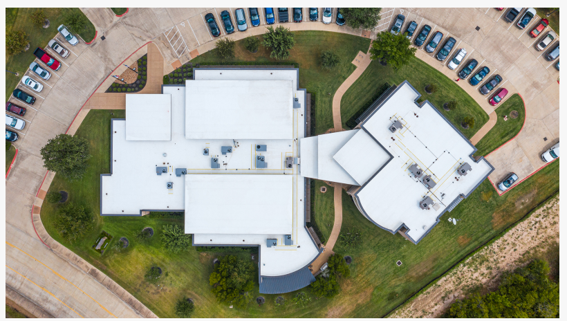
A drone capture of a completed roofing project.
