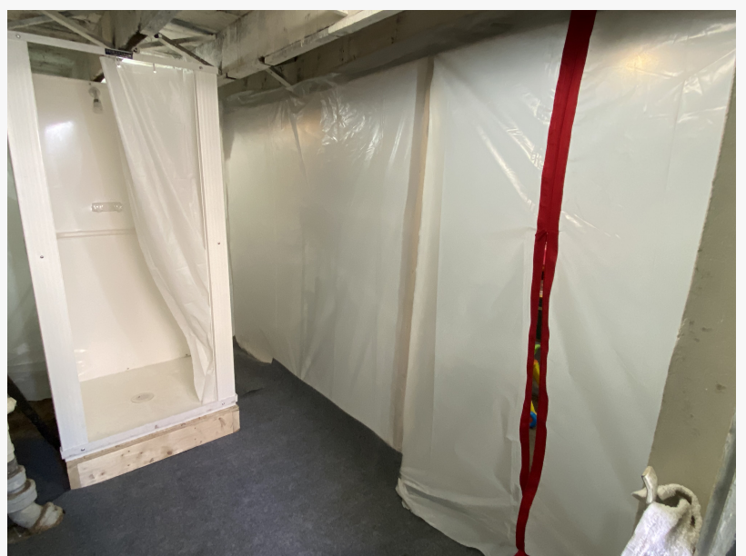
The Temporary Shower Installed in the Basement
