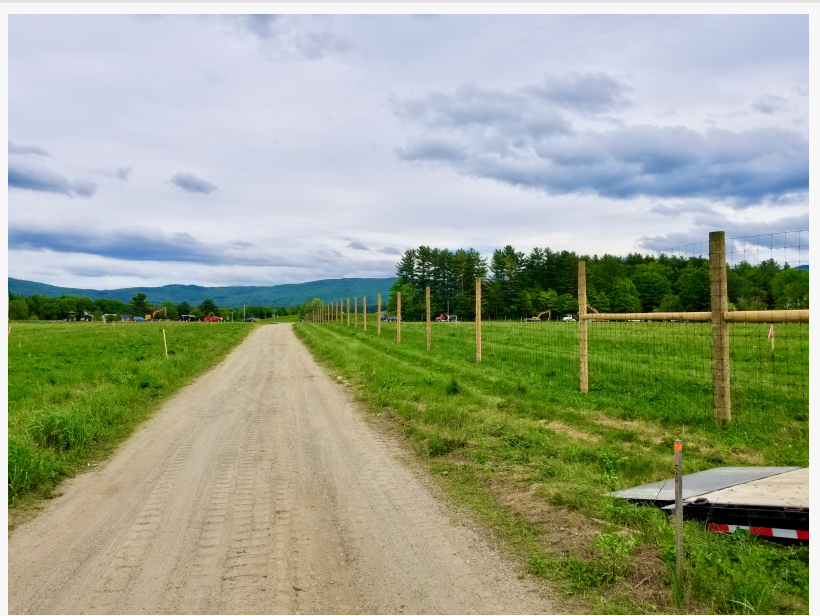
Construction begins on Lawrence Brook Solar
