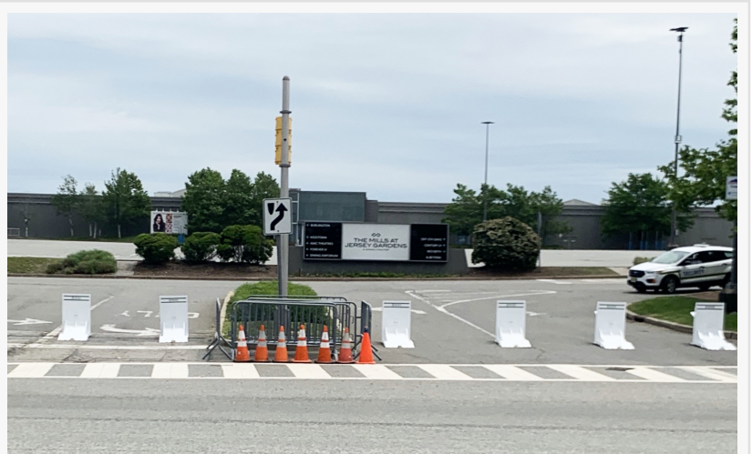
Meridian barriers protect Simon Mall location in New Jersey.
