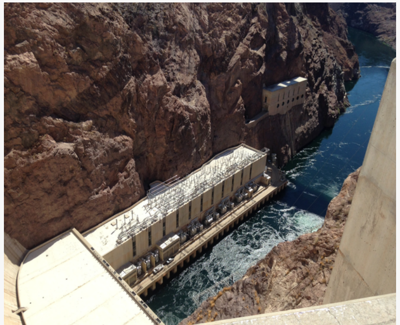
Hoover Dam Water Treatment Project - ICM
