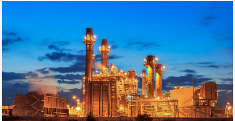
Power Generation Inspection and Safety Coordination
