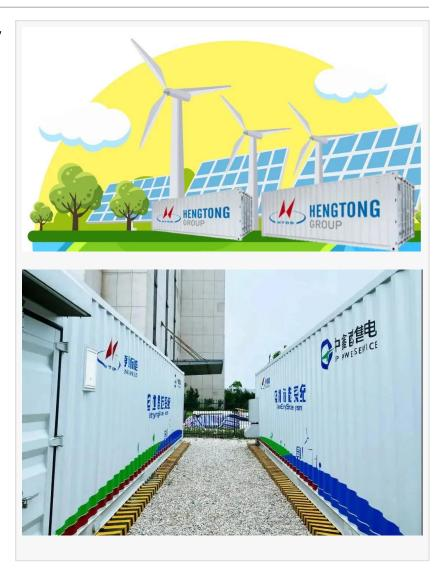
of thermal insulation, corrosion resistance, earthquake resistance and waterproof. The capacity of each container is 500kW/2MWh.
