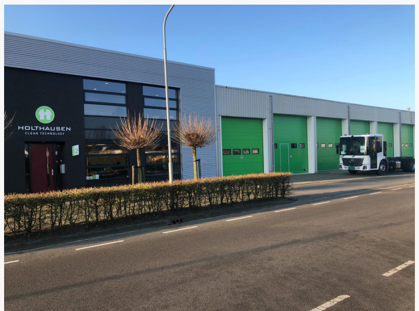
Integration Facilities in The Netherlands
