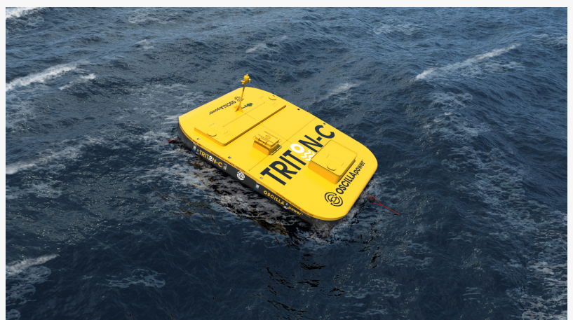
Aerial view of the Triton-C Wave Energy Converter
