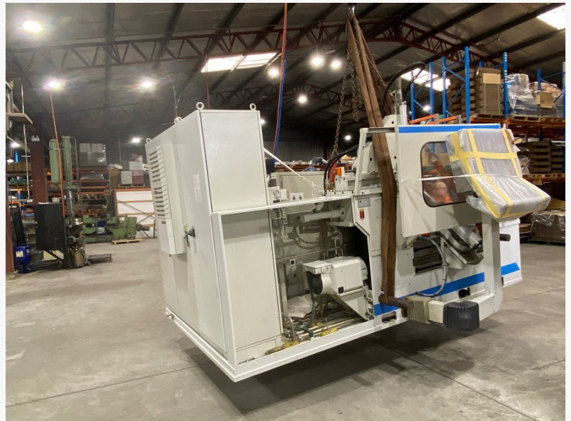
New Leifeld CNC Spinning Machine Being Installed
