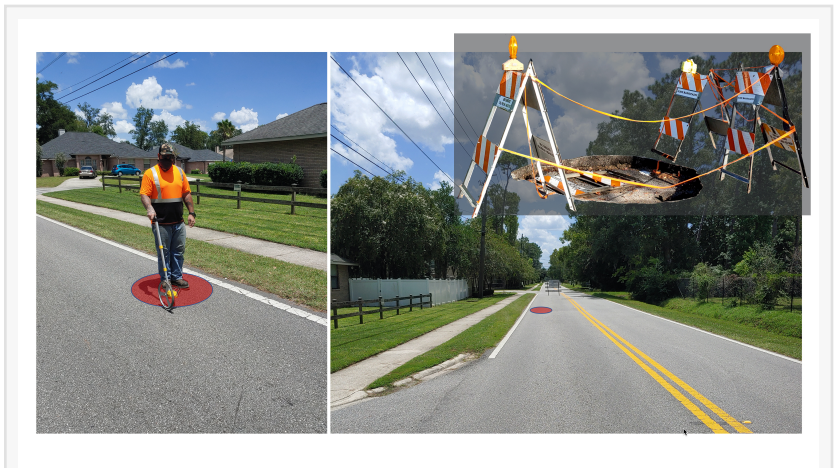
Electro Scan field crews match internal pipe defects with above ground subsidence to identify pre-sinkhole risk assessments.
