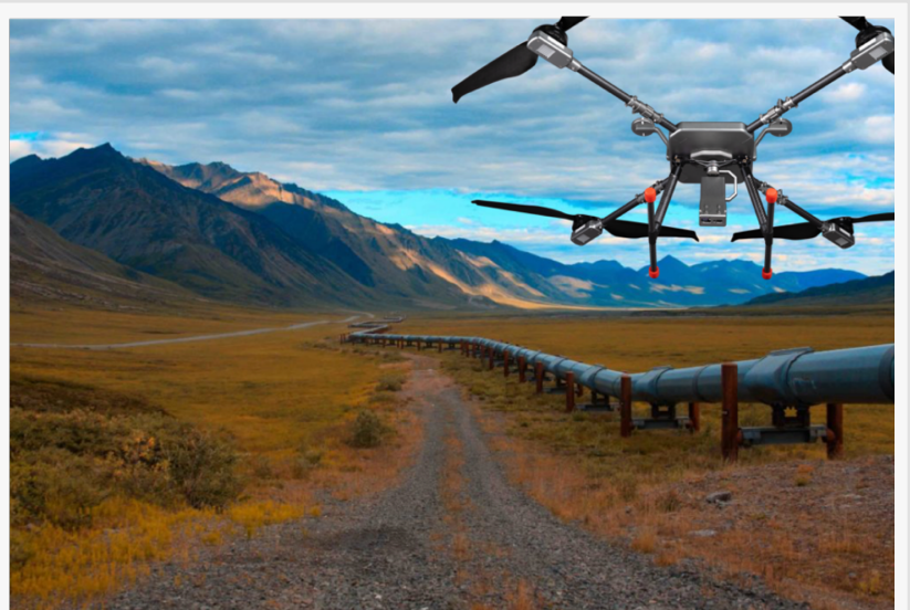
Methane Drone inspecting pipeline
