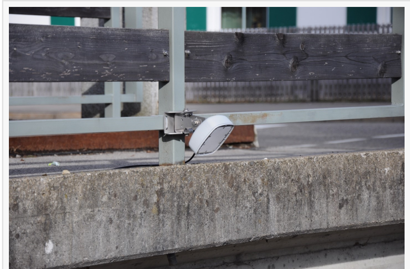
OTT SVR 100 installed in the field.
