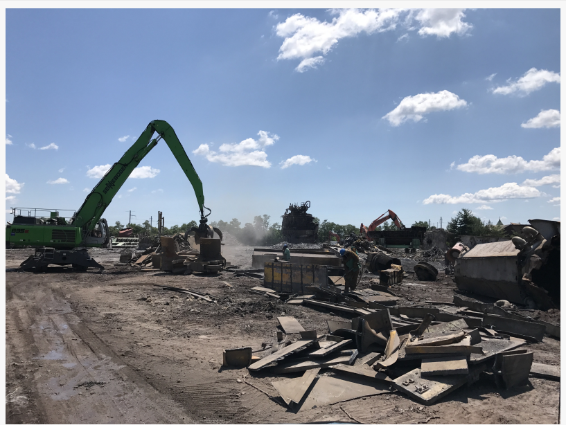
An excavator at work
