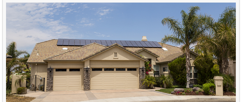
Solarize Solar Installation
