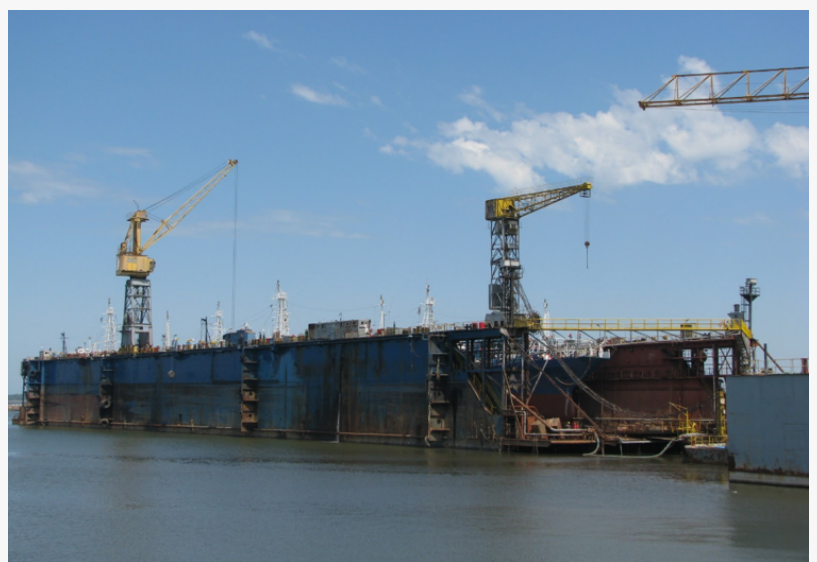
Floating dock side view. It is 220 yards long and 18 yards height from upper deck to bottom
