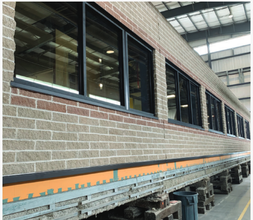
Modular Prefab Building being constructed in the factory
