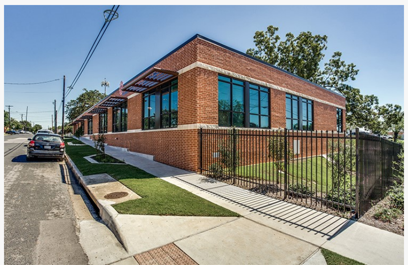
Brick Faced Modular Building
