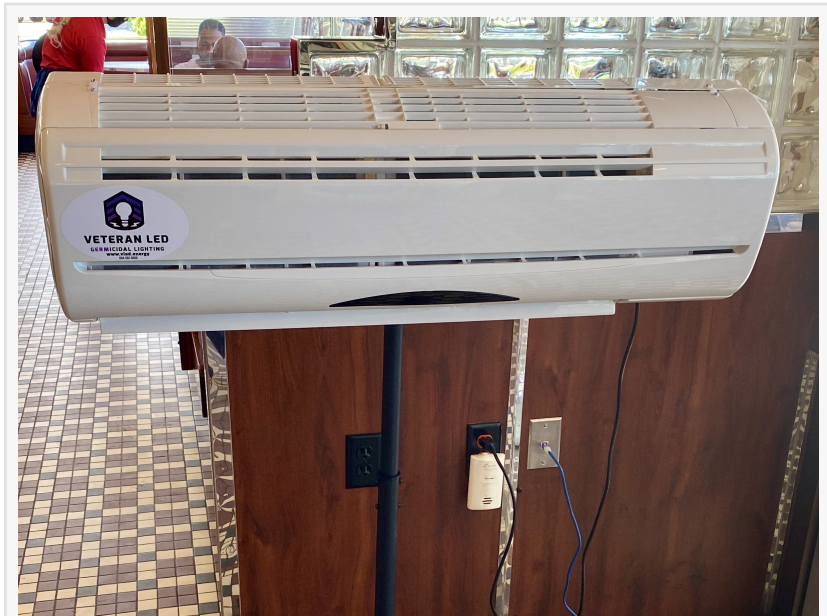
Large air purifiers with ultraviolet light and HEPA filtration are used in high-trafficked areas such as the hostess stand.
