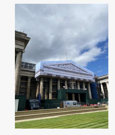
to be hung vertically, unlike debris netting which is usually installed horizontally. The sheets were finished with a pocket at the bottom for a scaffold pole to hold the sheet in place. Almost 50 panels totalling 2,800 square meters were used, making it one of the largest building wraps produced this year.
