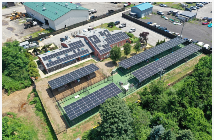
Commercial Solar System Installation
