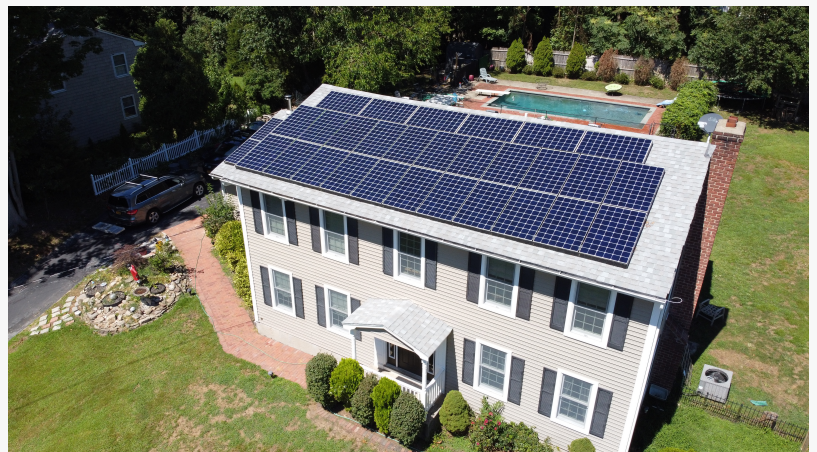
Residential Solar System Installation
