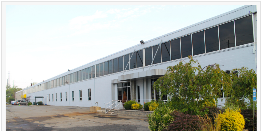
CRE Lending Group structured a $15 million refinancing package on this 377,000-square-foot warehouse in Kearny, New Jersey.
