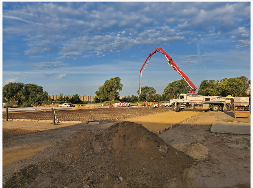
Pouring the foundation of Custom Dredge Works new Dredge Assembly Building.
