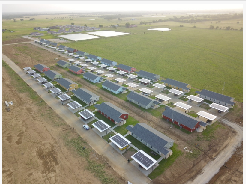
Sunview Homes and Sunfinity Renewable Energy created solar-topped carports for this housing development outside of Durant.
