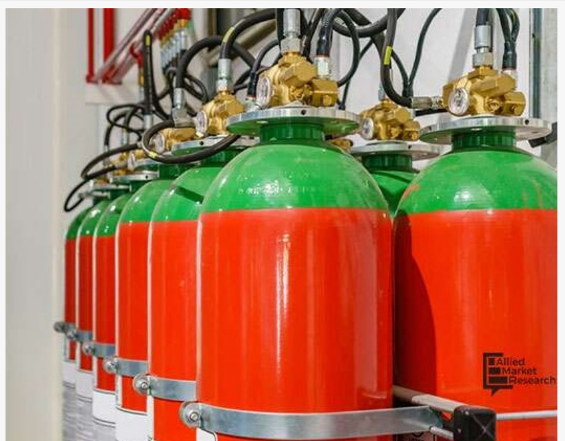
Fire Suppression Equipment
