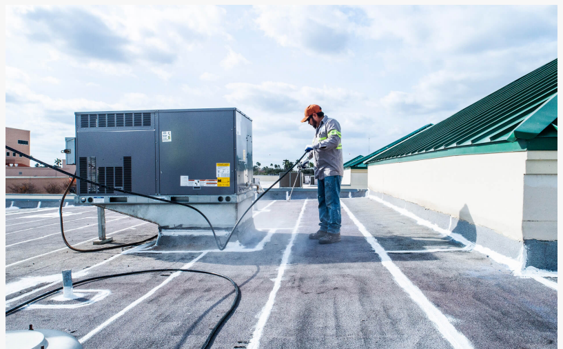
McAllen Valley Roofing Co. crew member spraying silicone on a commercial flat roof.
