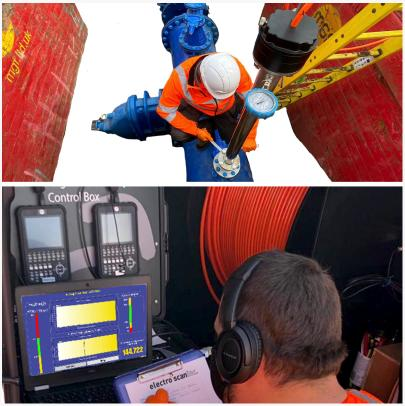
Electro Scan UK Team setting-up its intelligent probe in a pressurized water main.
