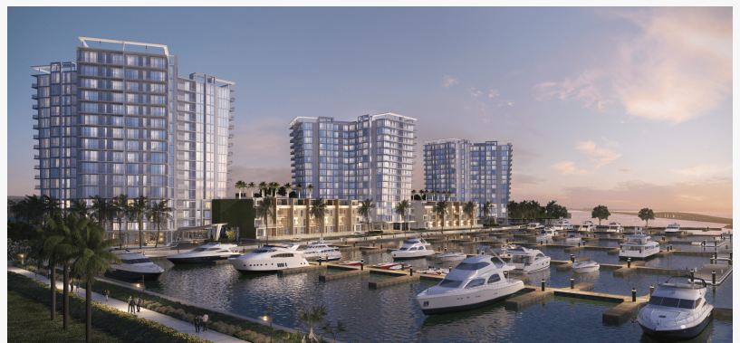
BTI Partners' Marina Pointe in Tampa
