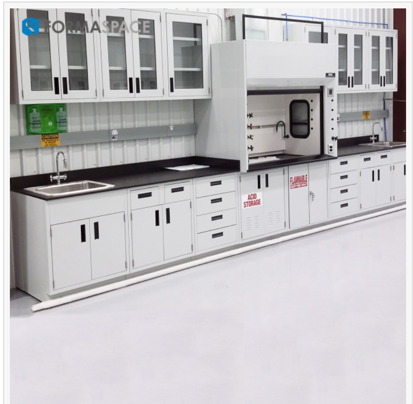
Formaspace manufactured the casework laboratory furniture for this Completion Science lab.
