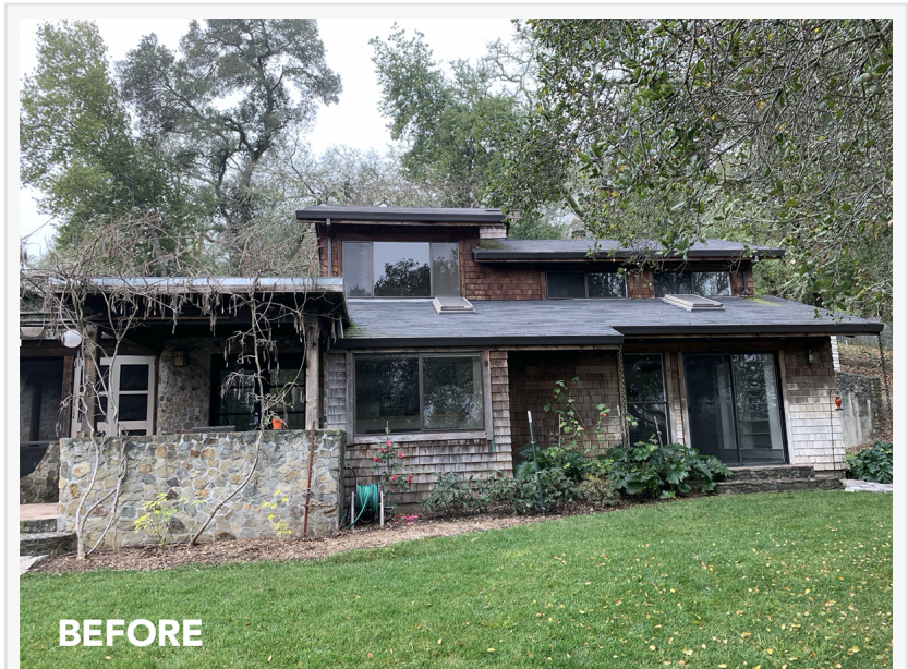
BEFORE image of the NARI Award-Winning Whole-House Remodel Project by LEFF Construction Design Build
