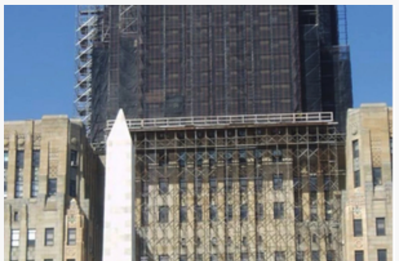
Scaffold Debris Netting
