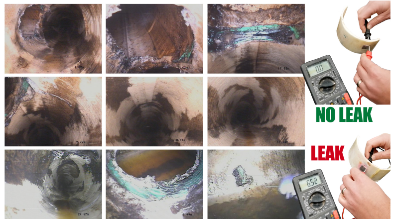
UK-based Cured-In-Place Pipe (CIPP) assessment project completed in 2020.
