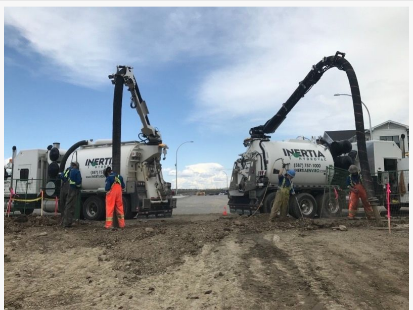
Inertia Hydrovac- Offers Dewatering & Jetting Services
