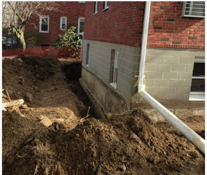
Drainage System Installation
