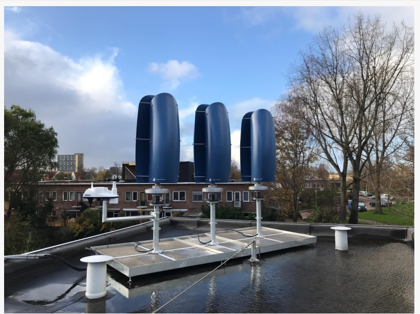
Flower Turbines Small Size Wind Tulip Installation
