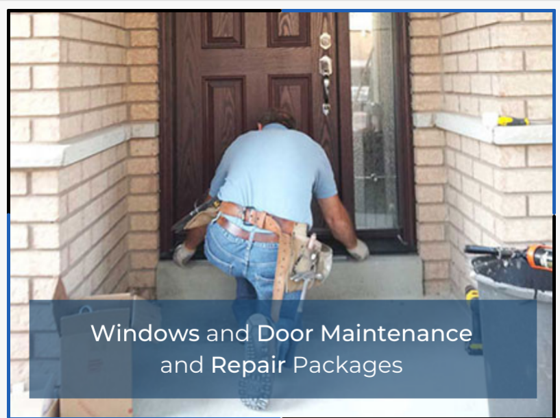
Windows and Door Maintenance and Repair Packages
