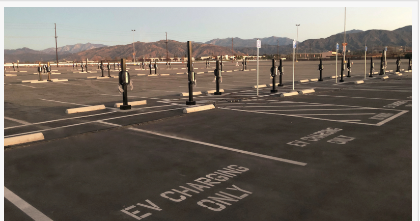
Rows of EVSEs on Fairplex main parking lot
