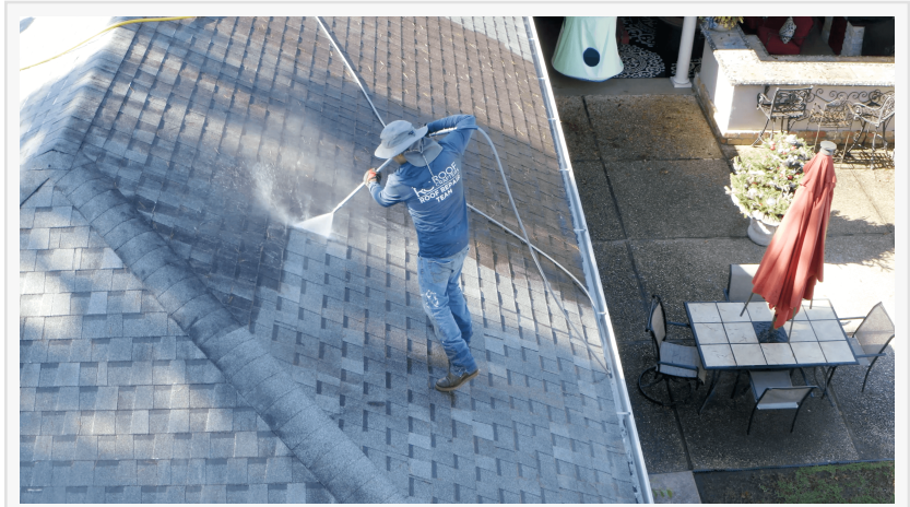
Roof Washing by Roof Crafters
