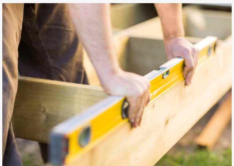
Worker Leveling a Deck
