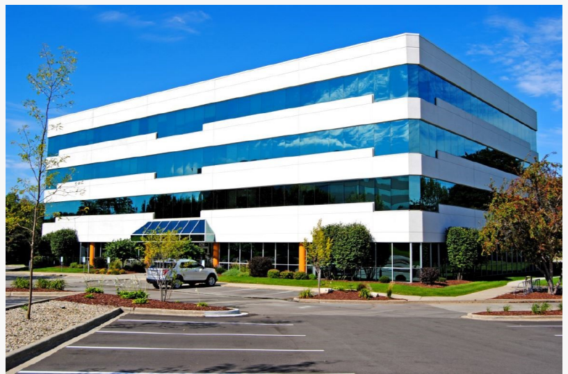
Park West II, located in Madison's University Research Park, is one of the Compass Properties buildings where the NPBI system was installed.
