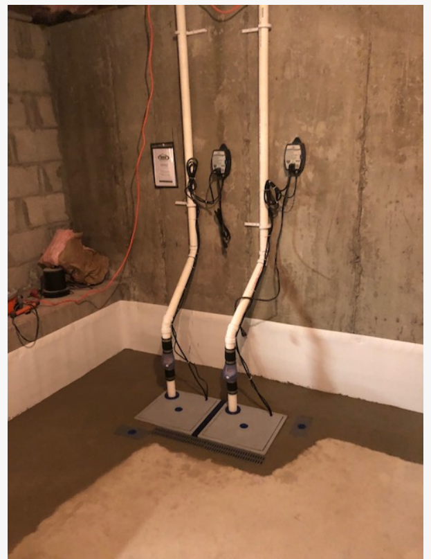
AFTER- Basement Waterproofing Services RI
