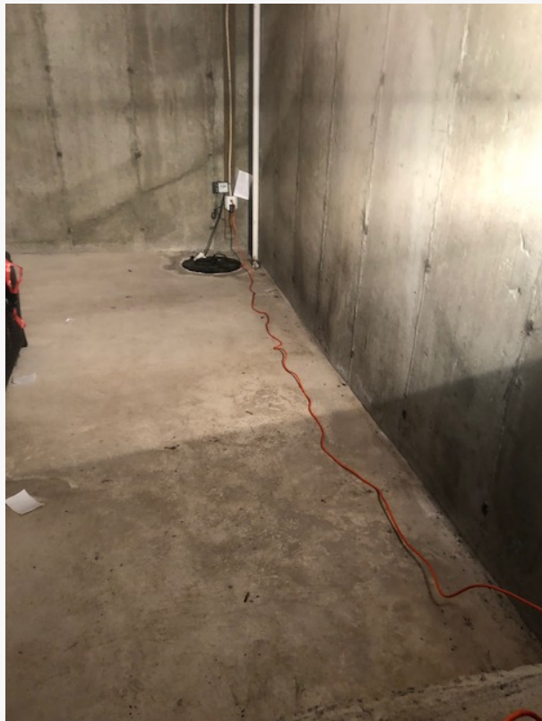
BEFORE- Basement Waterproofing Services RI
