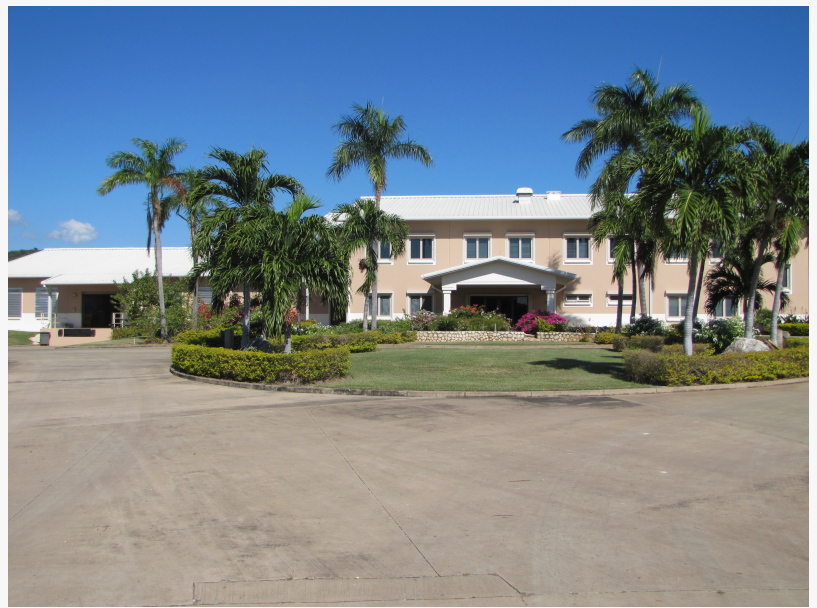
Marlie Technology Park Vidal Terrace Administrative Office Building
