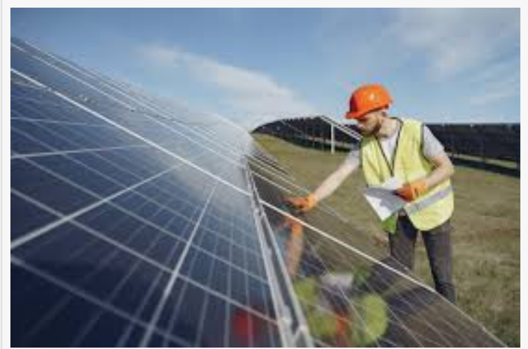
$SIRC work being performed
