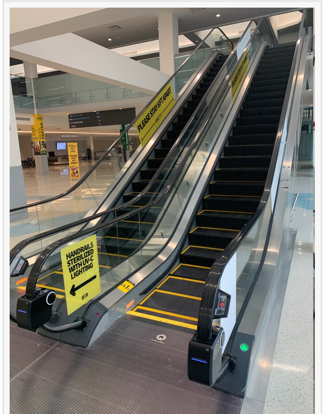
Clearwin UV-C Escalator Handrail Sanitizer installed at Syracuse Hancock International Airport
