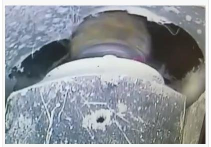
Customer service tap reconnection, frequently responsible for infiltration leakage rates greater AFTER rehabilitation, than BEFORE rehabilitation.
