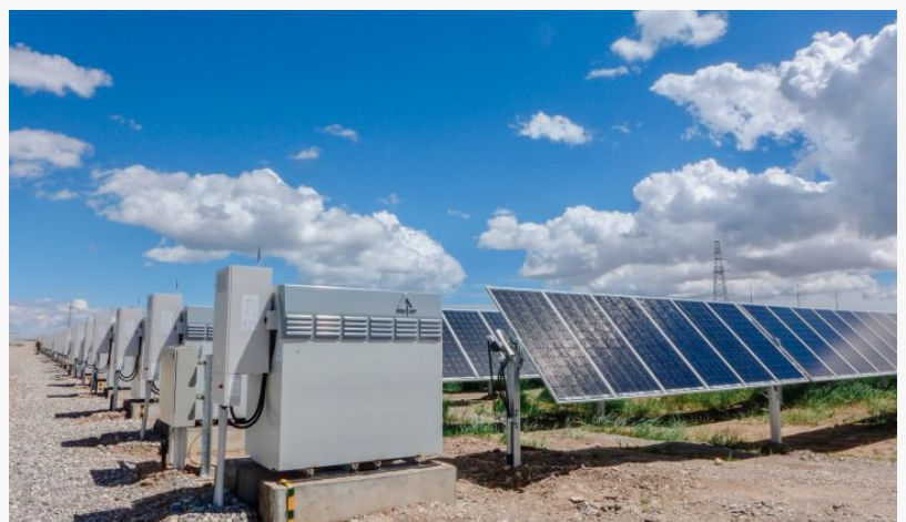
Vanadium Redox Flow Batteries supporting a solar energy installation. Photo courtesy of Invinity Energy Systems.
