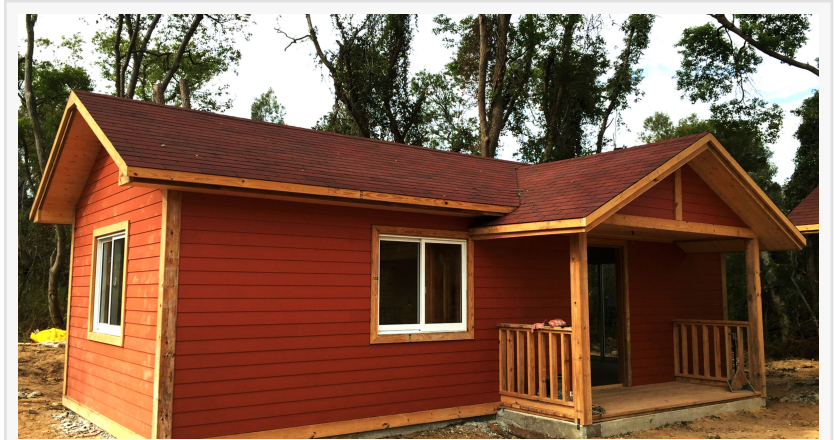
Building constructed through Plastic Waste Building Material (PWBM)
