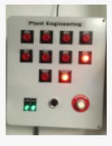
switches send an alarm signal over a Banner Engineering wireless network to an alarm cabinet in the boiler control room.
