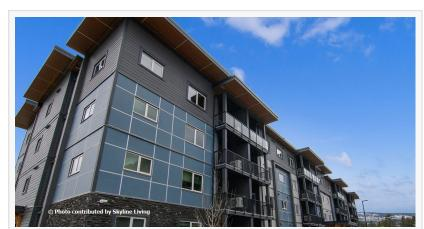
Carrington View Building A, a net-zero energy ready multifamily building, uses Insulspan SIP wall panels to create a tight building envelope. Photo contributed by Skyline Living.
